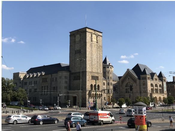
Fig. 3 Former Imperial Castle in Poznań, converted into Hitler's residence from 1939–1943 by Hans Böhmer and his studio, view from 2019
