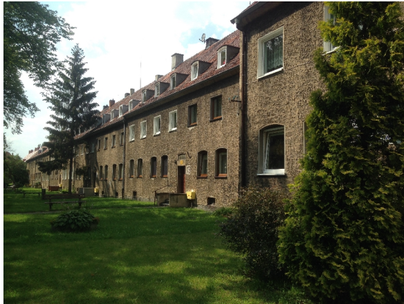
Fig. 6 Residential estate in Ostrów Wielkopolski, view from 2017
