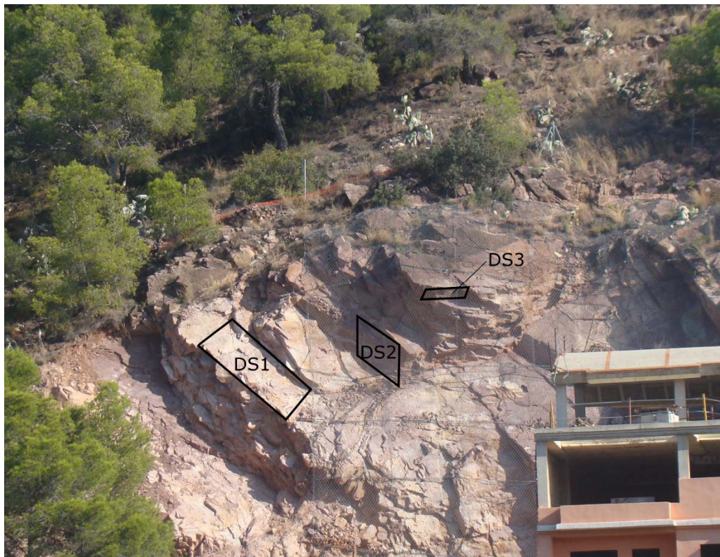
Fig. 14 – View of the slope of the example where three discontinuity sets can be distinguished.
