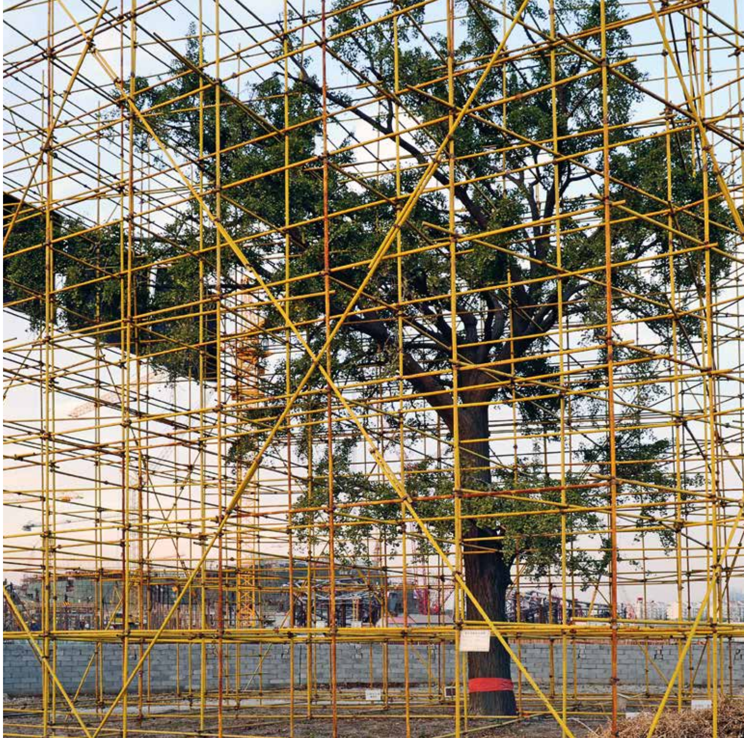
Construction side of new Shanghai Swimming Center, Pudong
