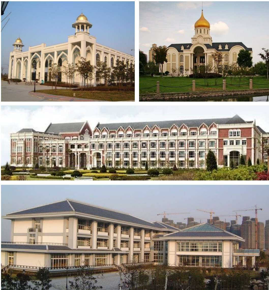
Figure 3.21: Departmental buildings of the Shanghai International Studies University
