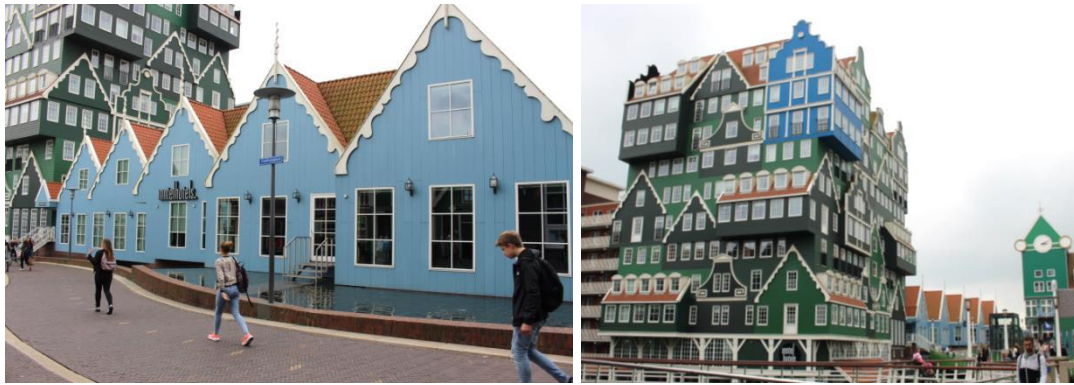
Figure 4.25: Inntel Hotel – the terraced-like units (left) and the main building (right)
