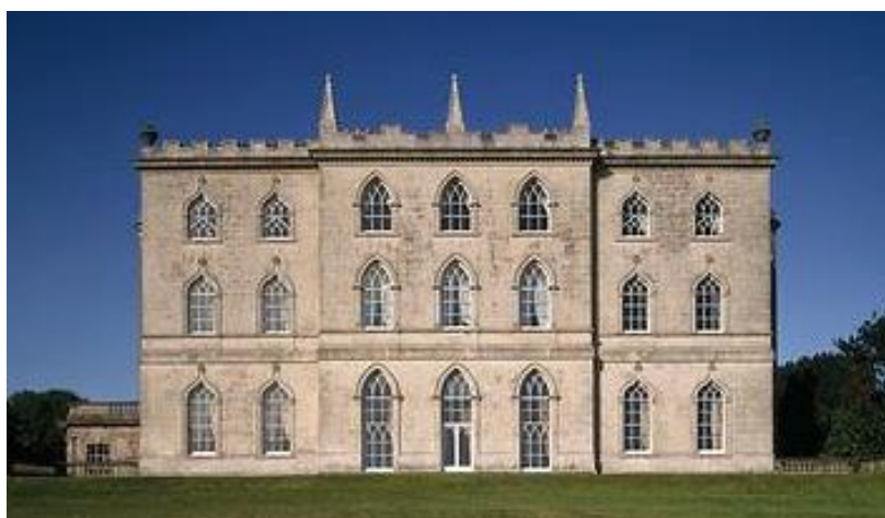
Figure 1.10: Classical and gothic façades of Castle Ward in Northern Ireland (1763)
