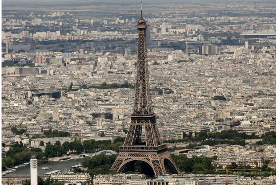
Figure A.3: Eiffel Tower in Paris, France (1887-1889)
