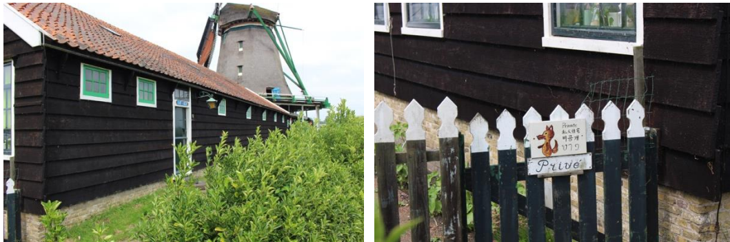
Figure 4.39: De Zoeker oil mill – private residence
