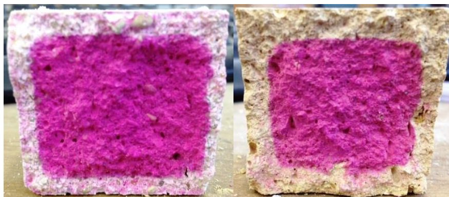
Figure 9. Phenolphthalein staining at 28 days
