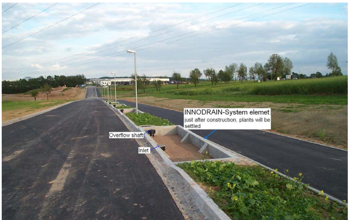
Fig 29. INNODRAIN-Elements along a transport road in Röhrsdorf Chemnitz, Germany
