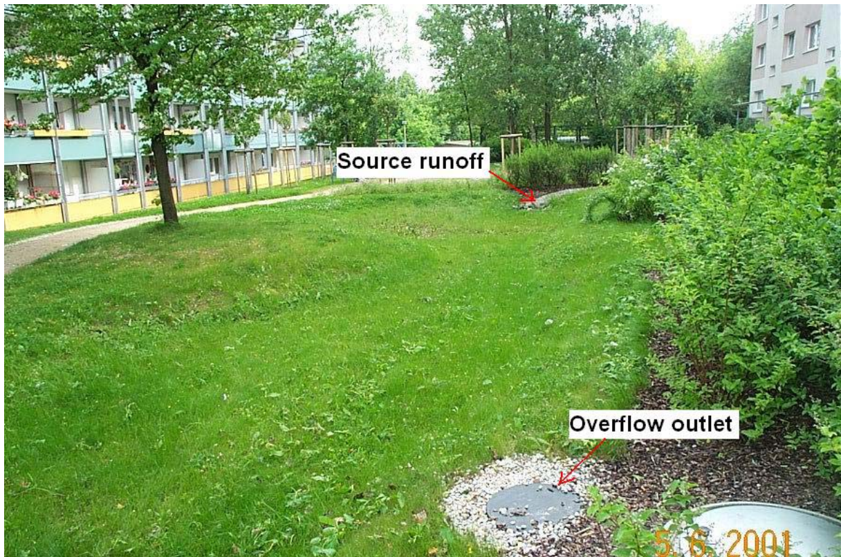
Fig 28. A Swale-Trench element in residential area Fritz-Heckert, Chemnitz, Germany
