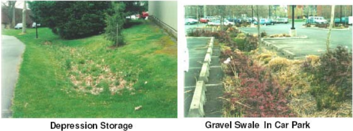
Fig. 1 On-site stormwater management measures applied in Auckland, New Zealand (source: On-Site Stormwater Management Manual Auckland City, 2004)
