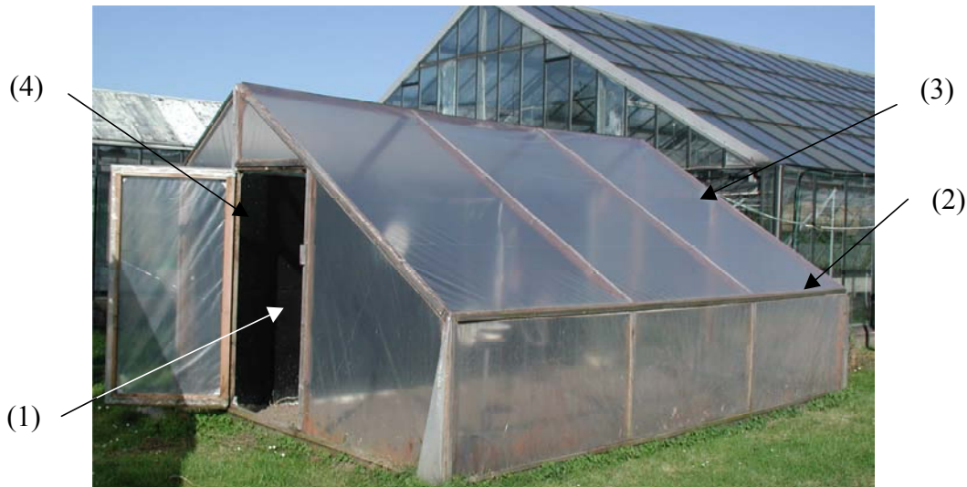
Fig. 5. 2. Greenhouse construction (1) concrete north wall and east-west gable, (2) construction material, (3) roof covering material and (4) greenhouse door.
