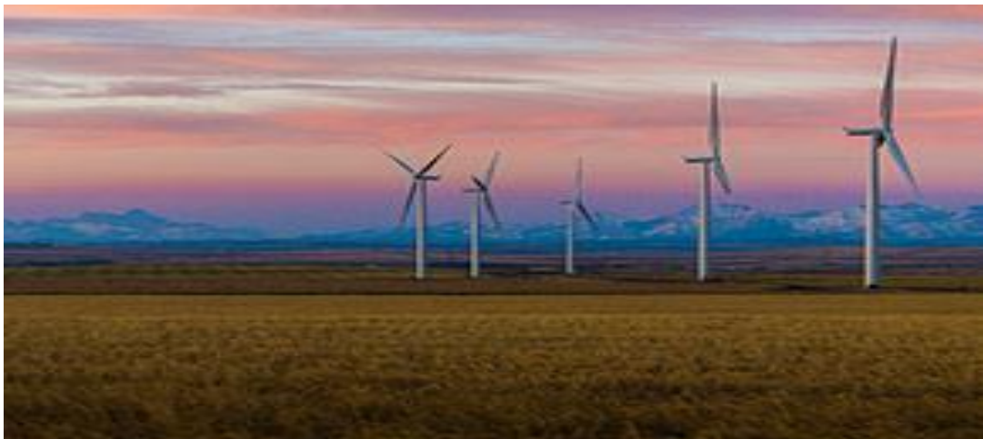
Figure 2.2. Onshore wind turbine.[5]
