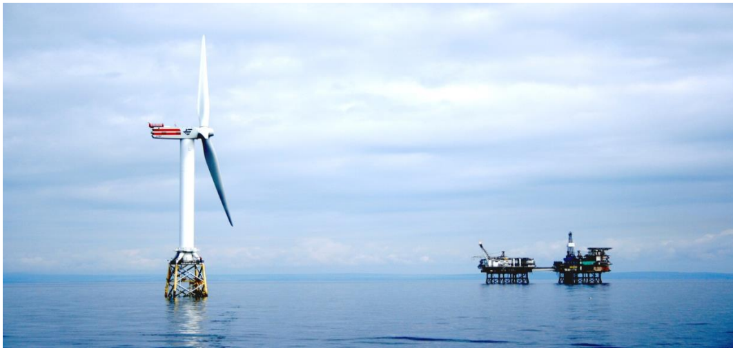
Figure 2.1. Offshore wind turbine (5-MW, 126m tall, 45m depth) Scotland.[7]
