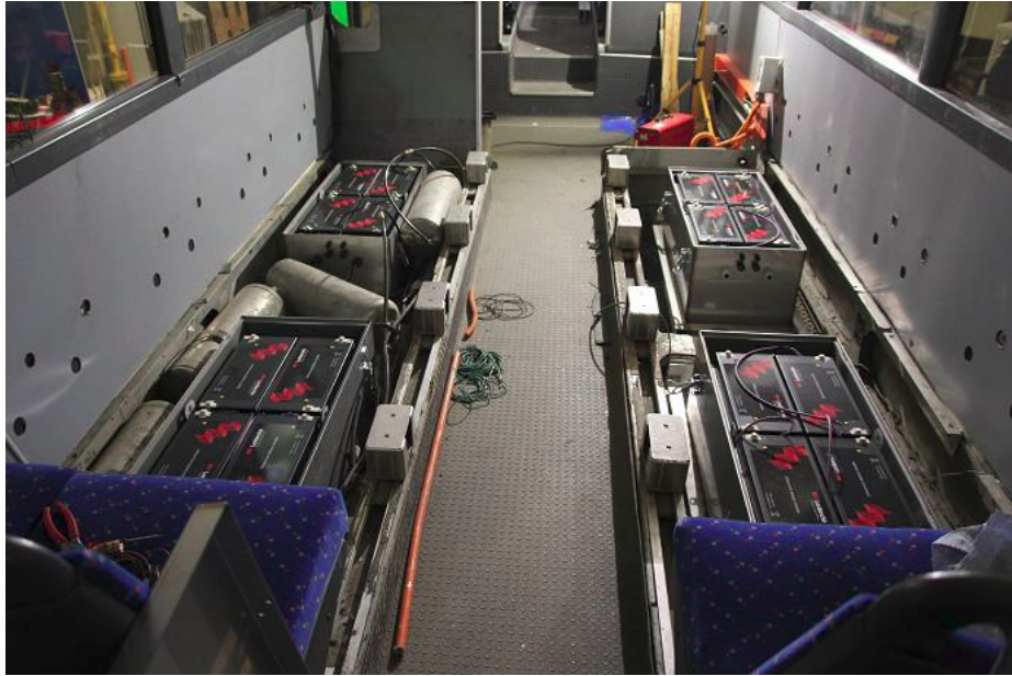
Figure 43. Leclanché LTO battery packs at the front cabin (VTT, 2016)
