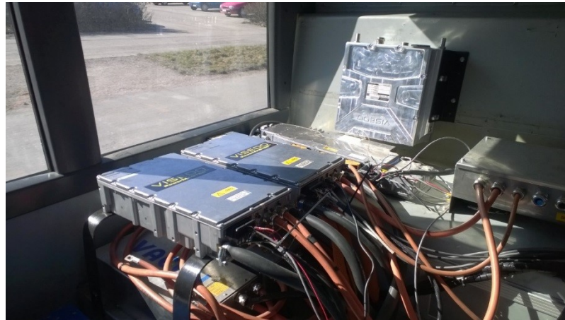
Figure 38. Inverters for PMSM (left) and auxiliary compressors (right)
