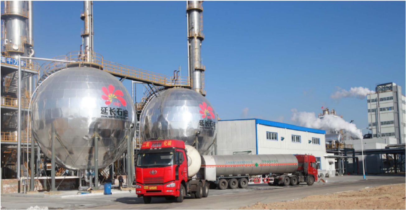
Figure 6-2 Yanchang Yulin Coal Chemical's 50,000 tonne Carbon Capture Facility
