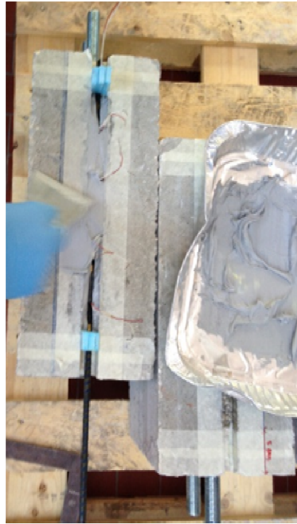
Figure 5b. Placement of thixotropic resin in the groove
