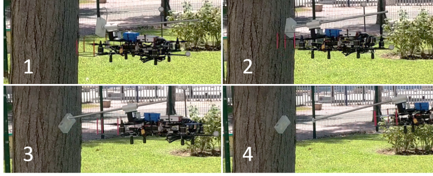
Figure 20: Time-lapse sequence of an aerial installation of sensor outdoors.
