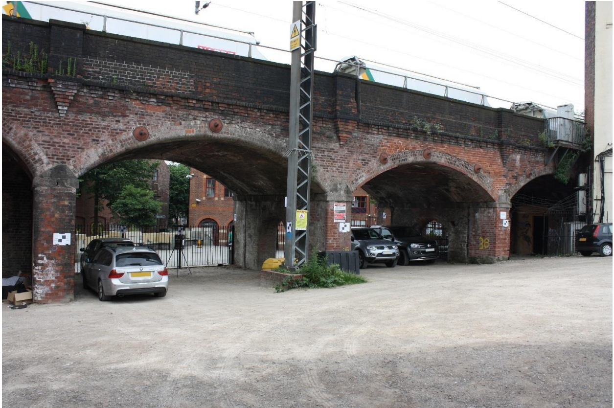
Fig. 2. View of the Marsh Lane viaduct
