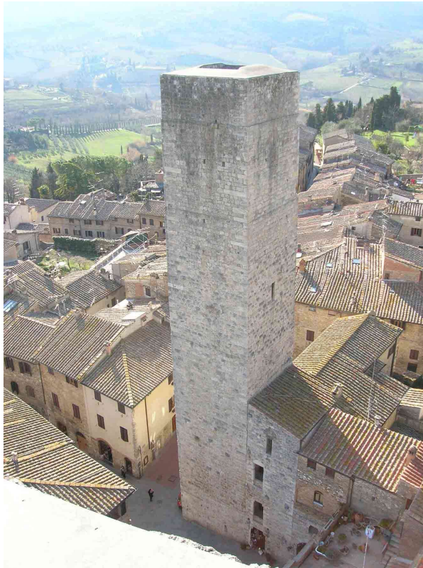
Figure 1 North-East aerial view of the Cugnanesi tower.
