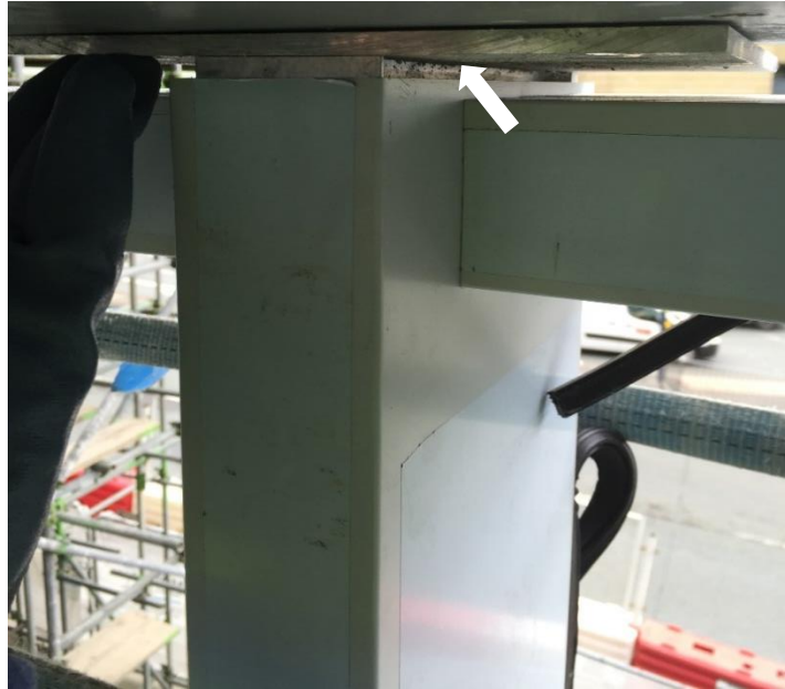
Figure 4-16. Adjustable connections for curtain walling
