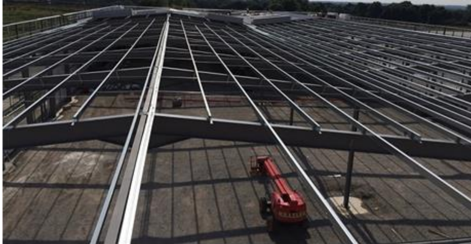
Figure 4-37. Installed purlins on the roof
