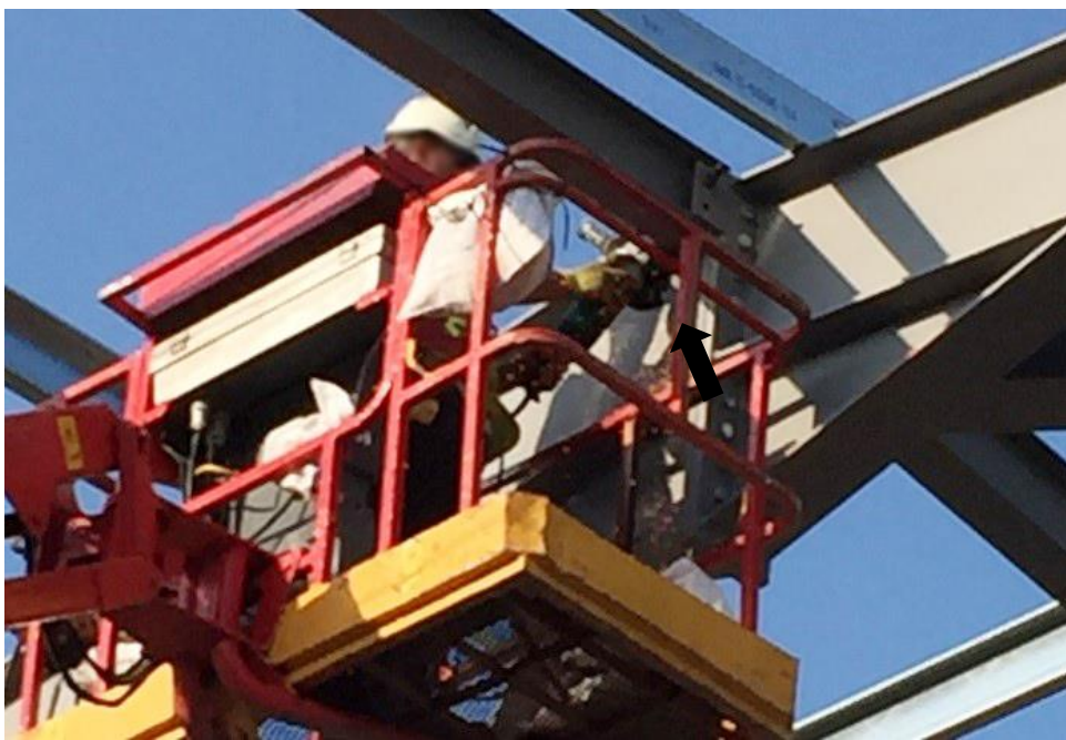
Figure 4-51. The steel erector trimmed the beam
