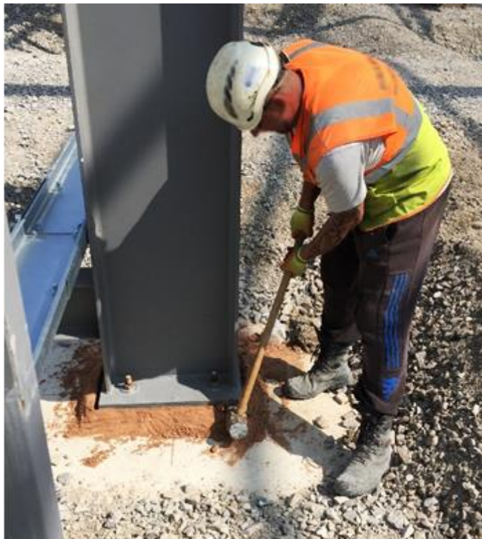
Figure 4-34. Steel erector adjusts the column using a hammer
