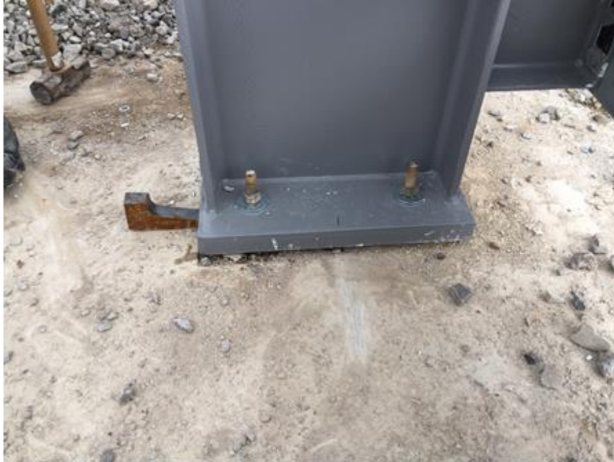
Figure 4-30. Wedging the column to fix it after being plumbed and levelled
