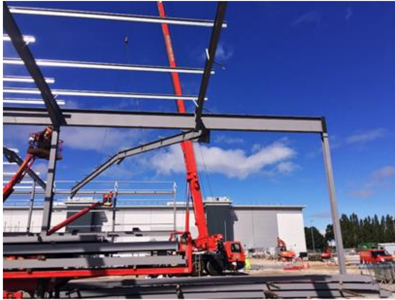
Figure 4-41. The crane inside the building up to Gridline 30
