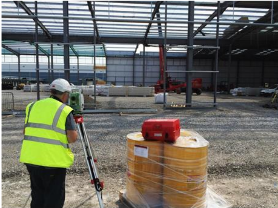
Figure 4-31. Location of the site engineer when measuring the misalignment of doorways
