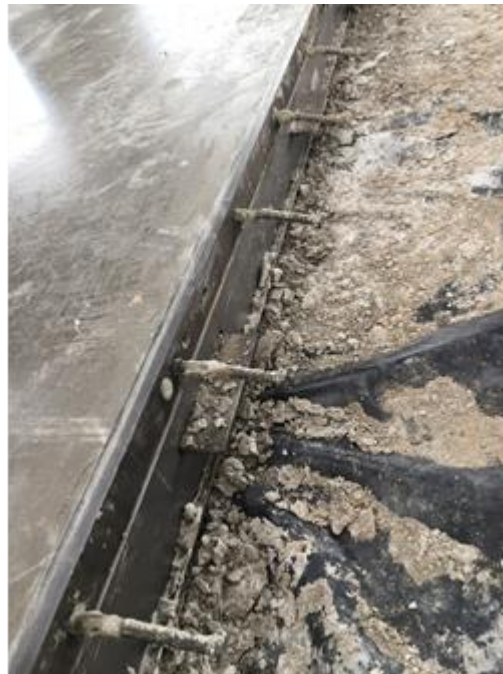
Figure 4-26. Butt connections for the interior concrete slabs
