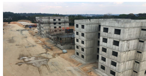
Fig.3: Construction site for residential buildings
