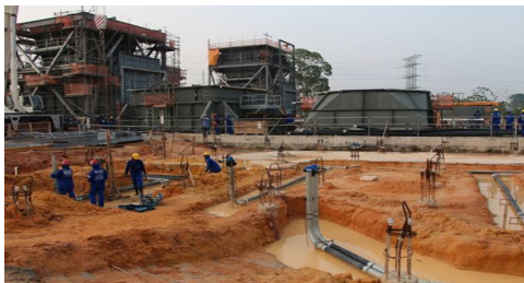
Fig.2: Construction Site of a Thermoelectric Plant
