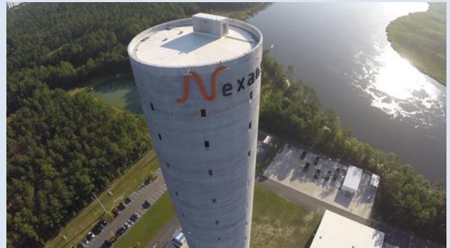
Pictured: The Nexans CVC Tower in Charleston
