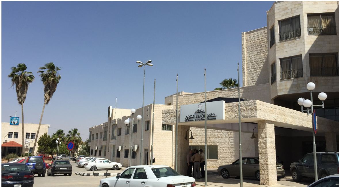
Figure 4. Ar Ramtha Hospital, Jordan. Photo: Andreas Älgå
