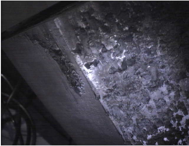
Fig. 45. View of part of the apron of a Tile 1 (right-hand side) and the upper front face of the tile (towards the left-hand side) during the 2007 JET shutdown inspection, showing spalling deposits. The tile had been exposed 1998–2007.
