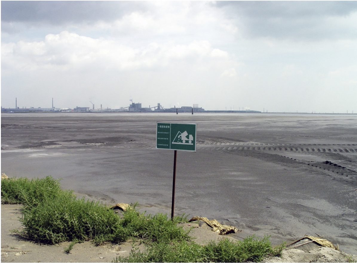
Figure 2.12: Photograph of the Baotou tailing dam [Li et al., 2013]
