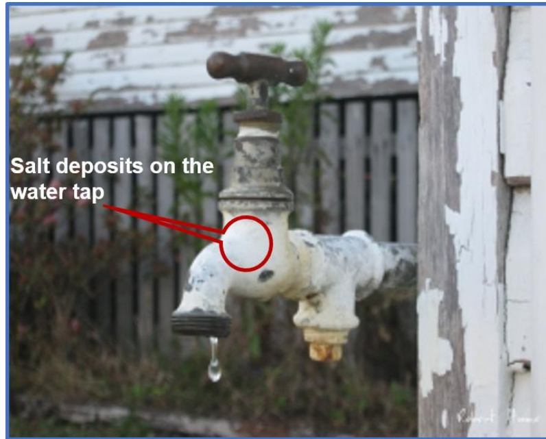
Figure 1.1: A picture showing public water tap with a salt deposit in Limpopo Province, South Africa (55,56).
