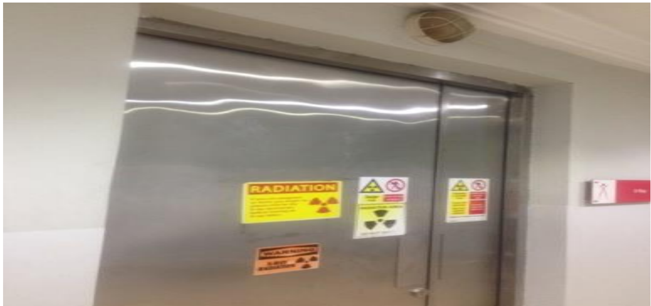
Plate 2: View of warning light above the door with danger signs on the surface of the door.
