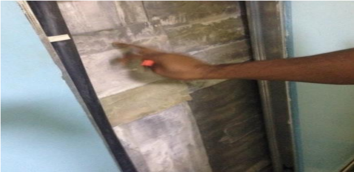
Plate 9: View of an uncovered lead lining in the 16-slice computed tomography room.
