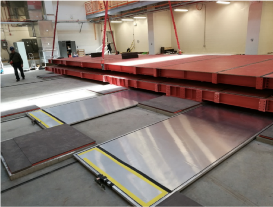
Figure 2.17: Picture of the currently installed Bottom CRT modules.
