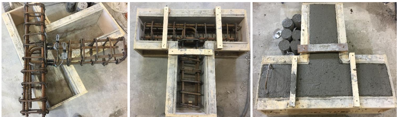
Figure 3-11 pouring of beam-column joints, formwork and reinforcement details
