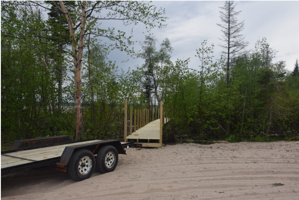
Appendix 1: Photo 8- The second boardwalk, closest to the river, under construction
