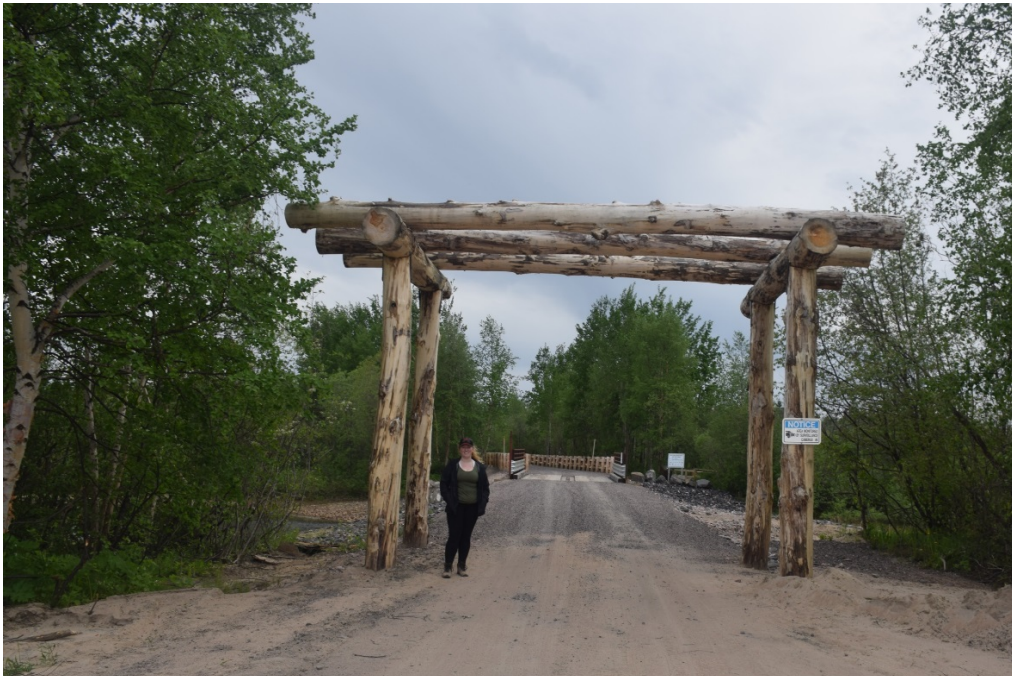
Appendix 1: Photo 5- The road entrance to Birch Island put in by HWL
