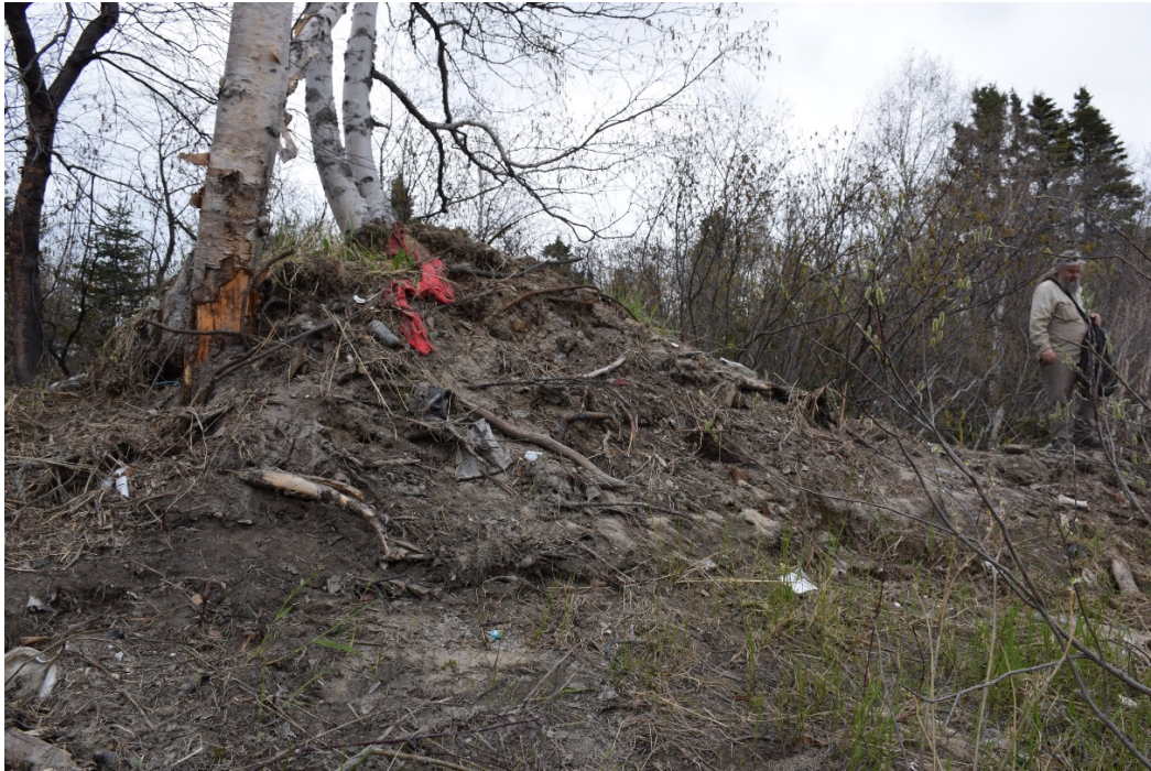
Appendix 1: Photo 23- Ice damage in the summer of 2017
