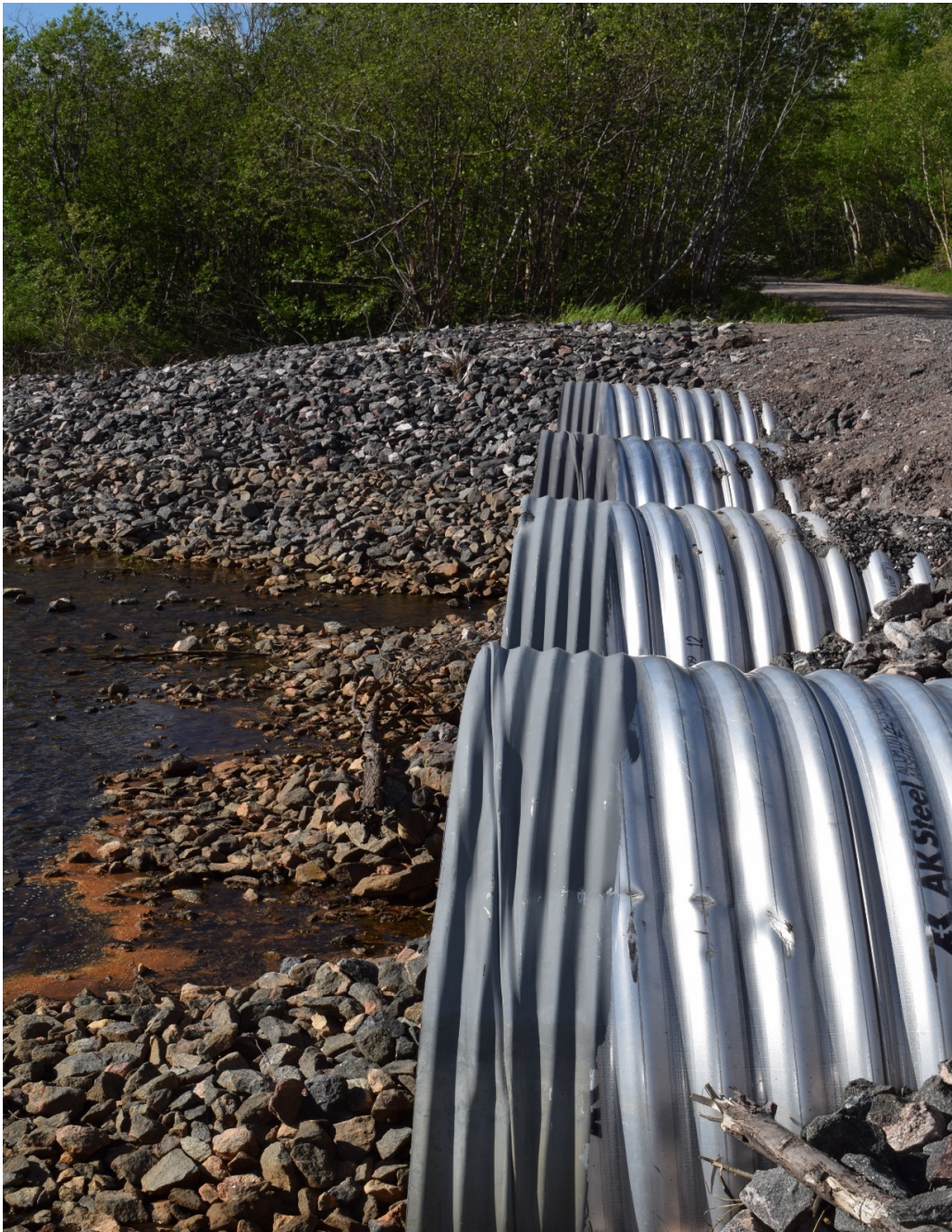
Appendix 1: Photo 1- One of two sets of culverts HWL replaced
