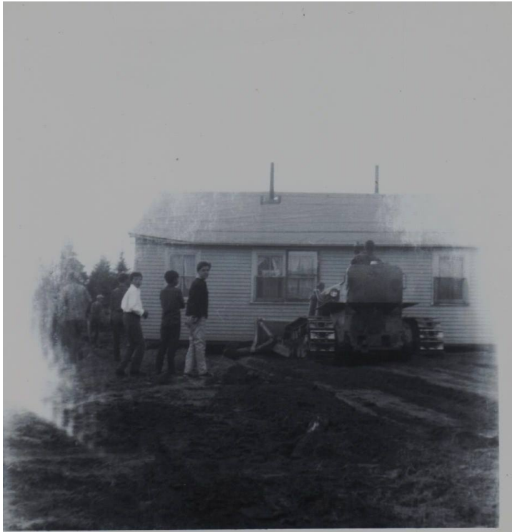
Appendix 2: Image 7- Moving a home off Birch Island during resettlement with a tractor (Courtesy of Henry Rich)
