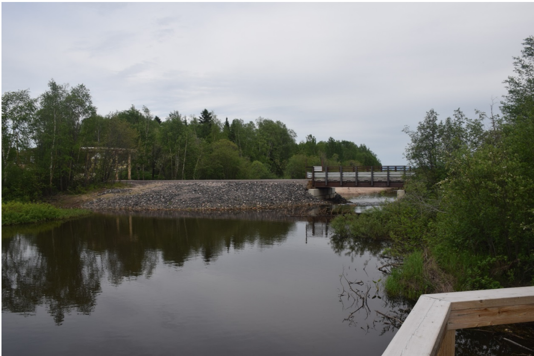
Appendix 1: Photo 3- Completed Construction on the Birch Island bridge.
