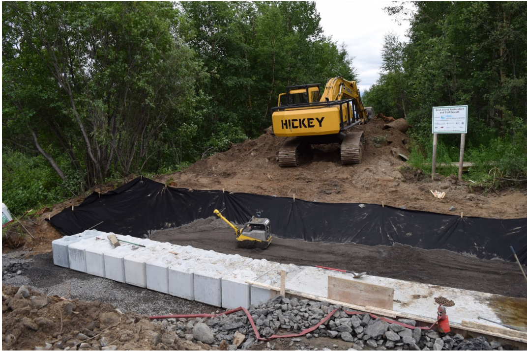
Appendix 1: Photo 2- Bridge construction over to Birch Island.
