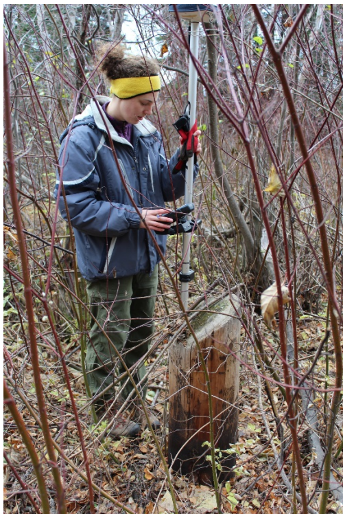
Appendix 1: Photo 22- Remnants of a telephone or electric pole on Birch Island
