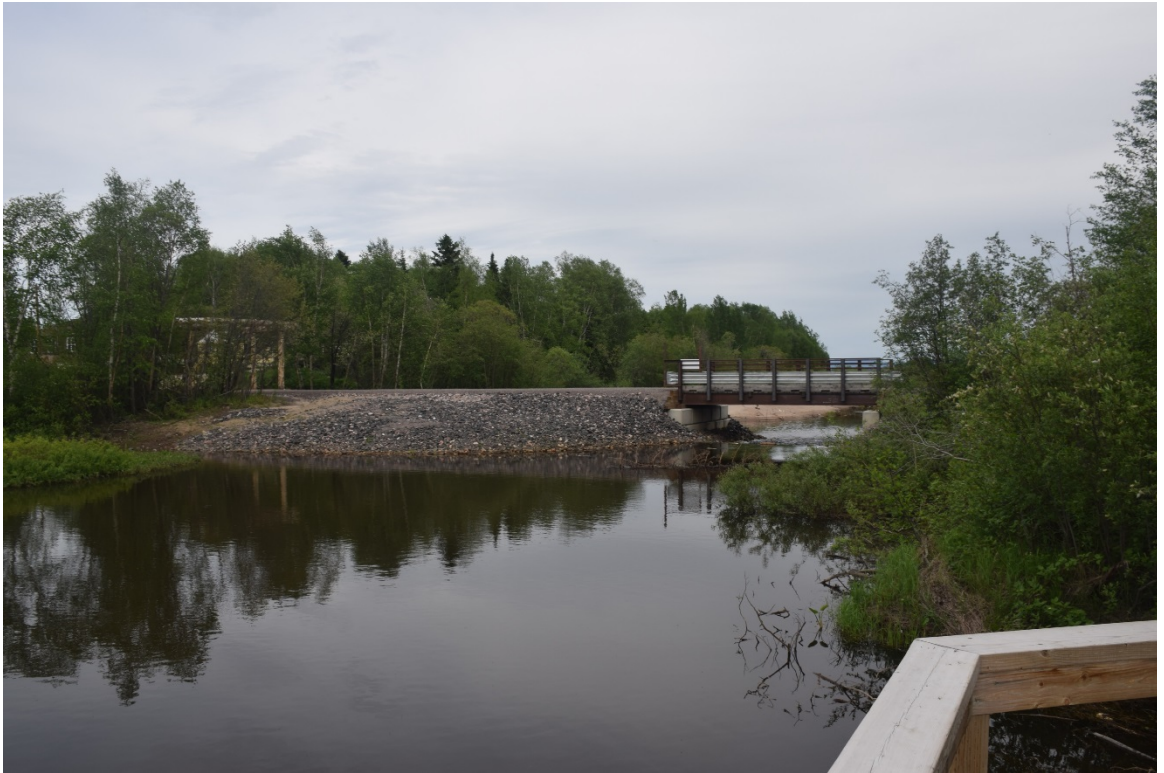
Appendix 1: Photo 61- Culverts replaced by HWL
