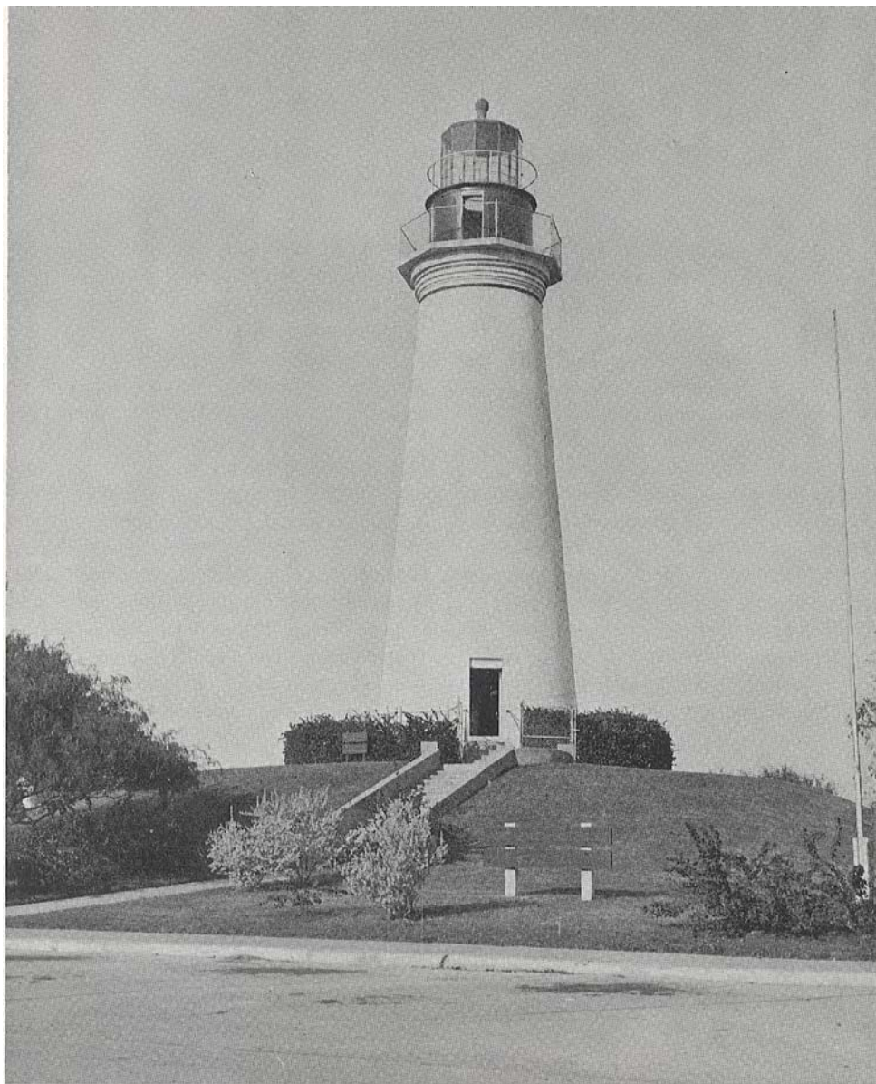
FIG. 93. Port Isabel Lighthouse. The only damage by Hurricane Beulah was four broken window panes. (Photograph by Texas Parks and Wildlife Department.)
