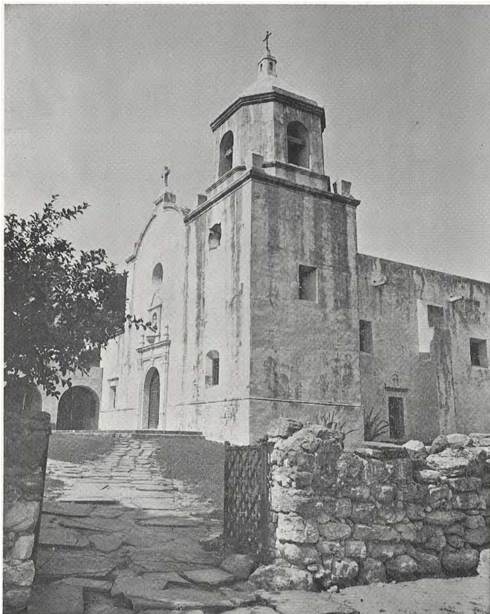
FIG. 63. Mission Señora del Espiritu Santo de Zuñiga at Goliad State Park. Stone in wall at gate to the mission is sandstone from the Goliad Formation. (Photograph by Texas Parks and Wildlife Department.)
