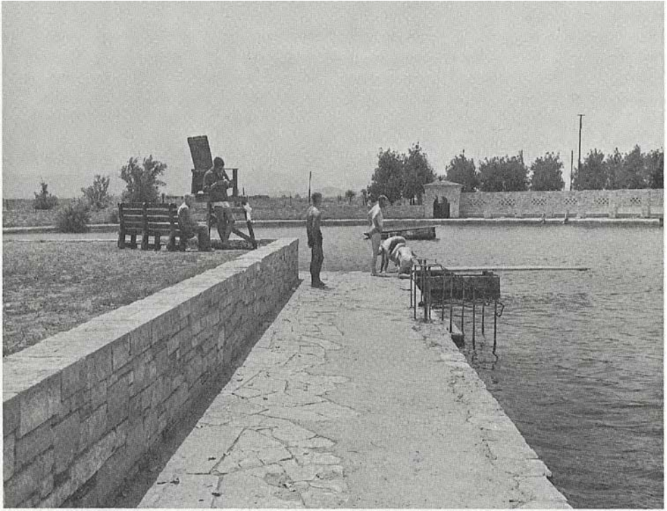
FIG. 25. The Balmorhea swimming pool which incorporates the total flow of San Solomon Spring. The spring was used by the Indians and frontiersmen and later for irrigation. Prior to the building of the masonry walls and walks of native Boquillas Flagstone, the water issued from a large swamp. (Photograph by Texas Parks and Wildlife Department.)
