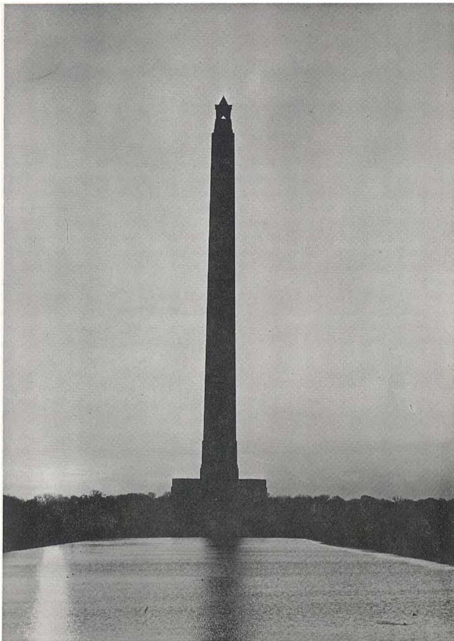
FIG. 96. Back lighting effect on San Jacinto Monument. This structure rests on a substantial foundation in the Beaumont Formation. Note the star near the apex of the monument. It is 35 feet high and weighs 220 tons. (Photograph courtesy of Texas Parks and Wildlife Department.)
