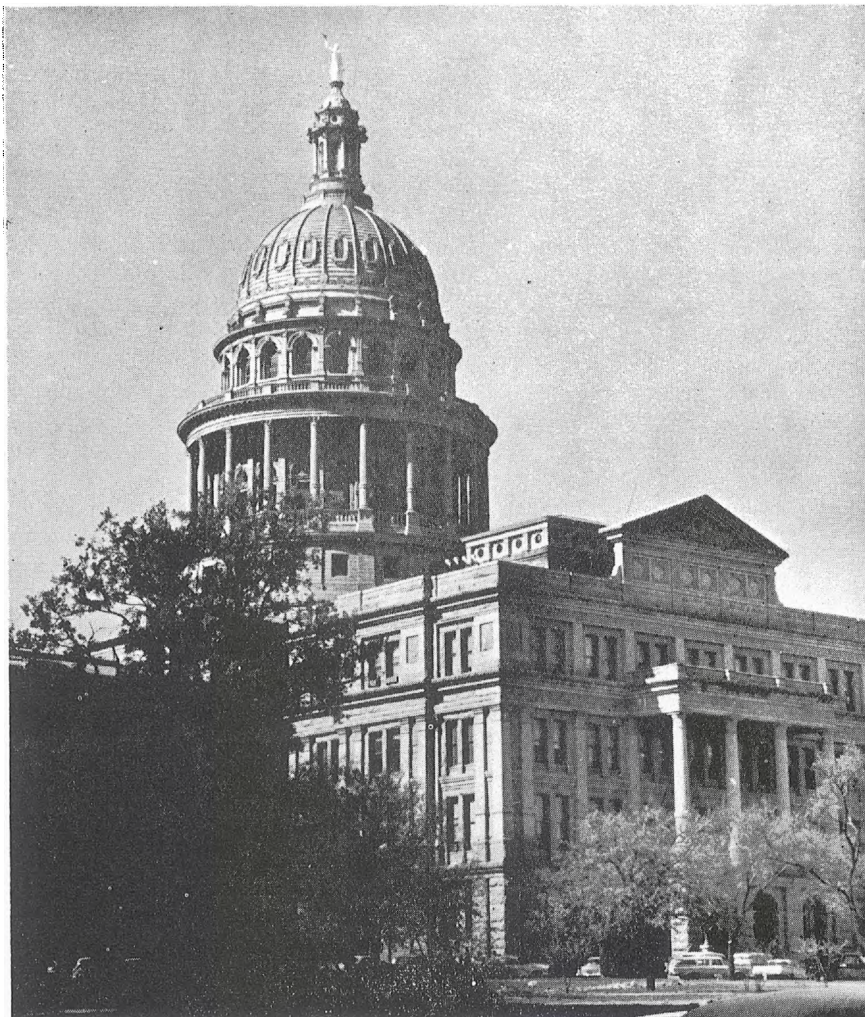
Texas State Capitol building at Austin is made of Burnet County granite obtained from Granite Mountain near Marble Falls, Texas.
