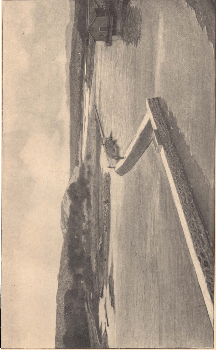
WING DAM OF EL PASO IRRIGATION COMPANY; LOOKING UPSTREAM.
