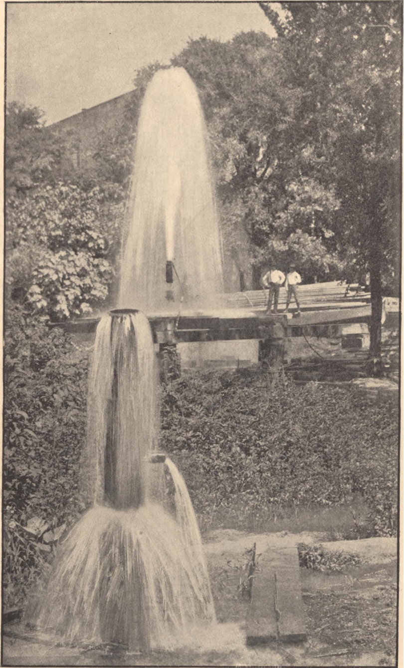
ARTESIAN WELLS AT CITY WATERWORKS, SAN ANTONIO.
