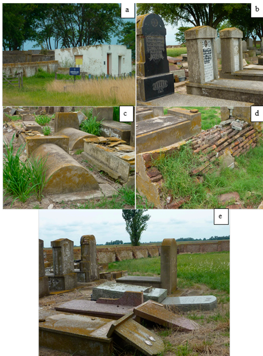
Figure 2. Conditions of the Algarrobo Cemetery: (a) view of the premises located in the front of the cemetery; (b) detail of tombs: stones with marble is observed; (c) view of the sector of the graveyard with tombs built in shape of vault; (d) detail of one of the tombs made with common ceramic bricks; and (e) view of some tombs affected by vandalism and the wall surrounding the cemetery.
