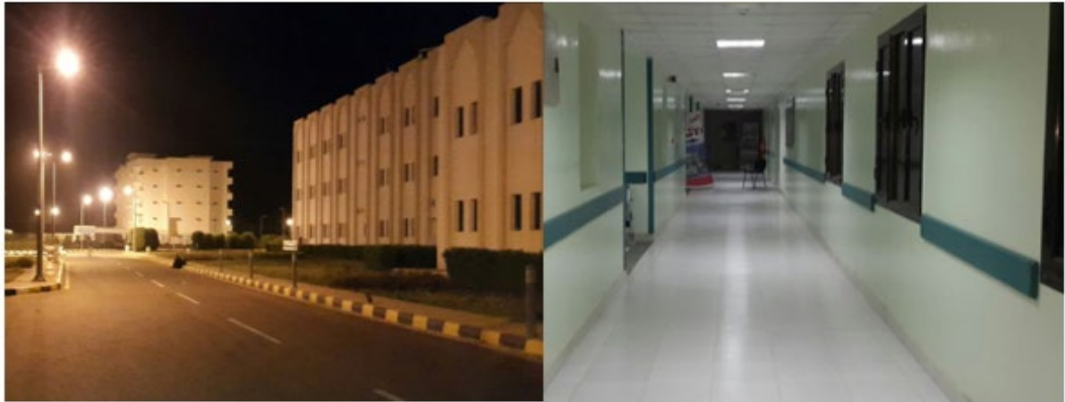
Figure 6.8 Merowe New Hospital (Chinese Hospital)
