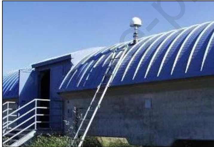
Figure 4. GNSS antenna mounted on the tunnel.
