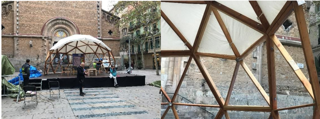
Installation of ESFERIC, Plaza de la Virreina, Barcelona
