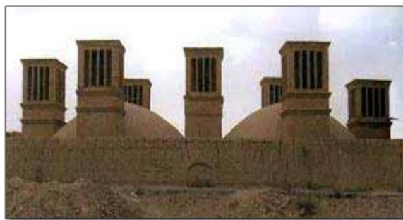
Fig .35 : A reservoir with two pools and seven Yazdi wind catcher in Hussein Abad close to the city of Yazd (by the author)
