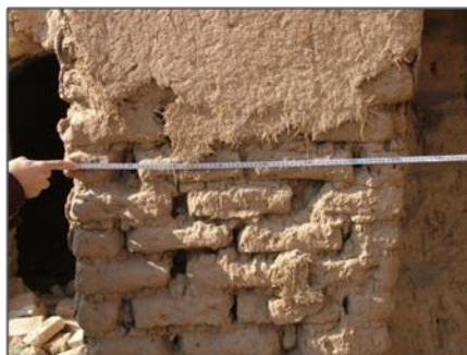
Fig .11: Thickness of traditional walls in hot and dry climate (by the author)
