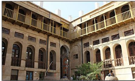
Fig .33: The central courtyard of the Kazerooni Seigniory, the current location of Bushehr's Cultural Heritage Organization (by the author)
