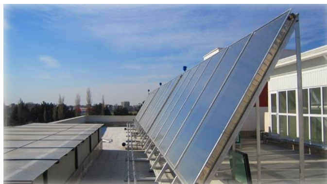
Fig .87: Use Solar Water Heater ( http://zero-energy.ir )
