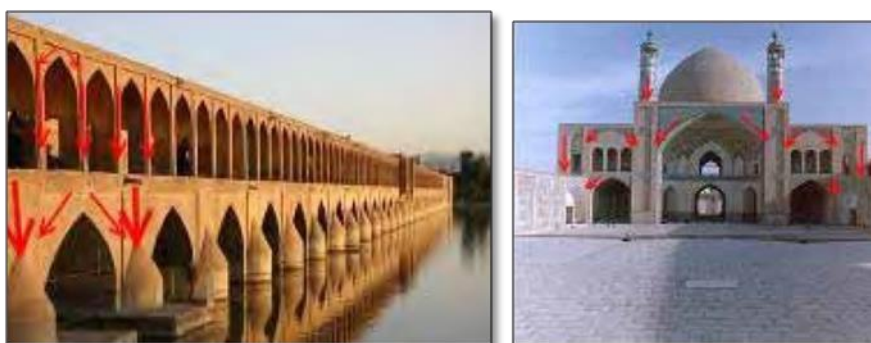
Fig. 32: Lightening the higher levels and spatial geometrics in domes and arches to endure the load (Qasemi & Geranmaye, 2013)
