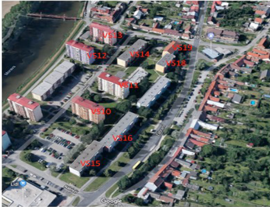
Fig. 2. An aerial view of the selected location
