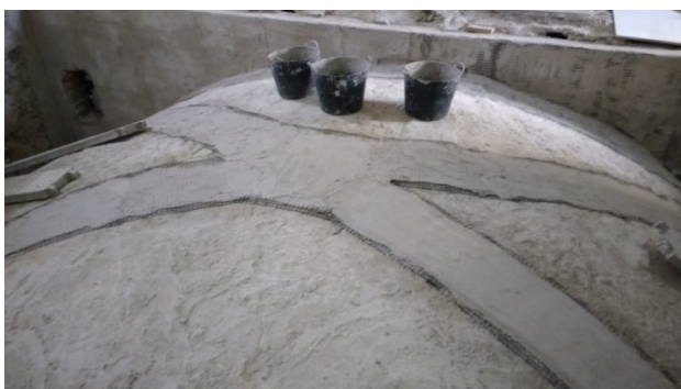
Figure 2: Reinforcement with Planitop HDM and fiberglass Mapei
