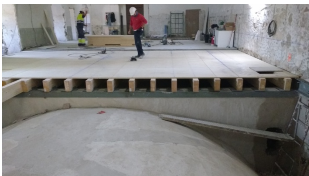
Figure 3: Reinforcement on wall ribs
