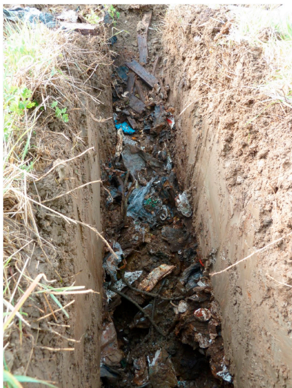
Fig. 3. Waste in Hadleigh Marsh flood embankment, trial pit 3.
