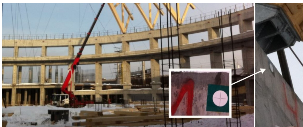
Figure 1. Fragment of ring beam and strain marks stuck on it
