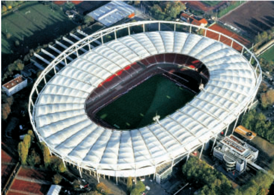
33. Spoked Wheel Roof covering the Gottlieb Daimler Stadium, Stuttgart, Germany, 1993.
