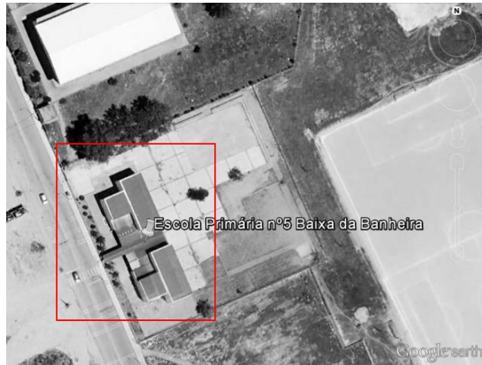
Fig. 2: General view of the school buildings and their orientation [26].
