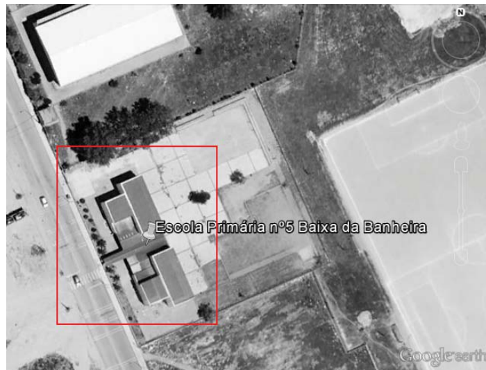
Fig. 3: General view of the school buildings and their orientation [10].
