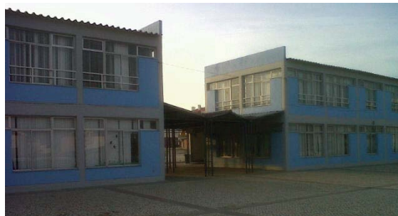
Fig.6: West view of the school.
