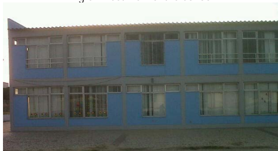
Fig.7: East view of one of the buildings.
