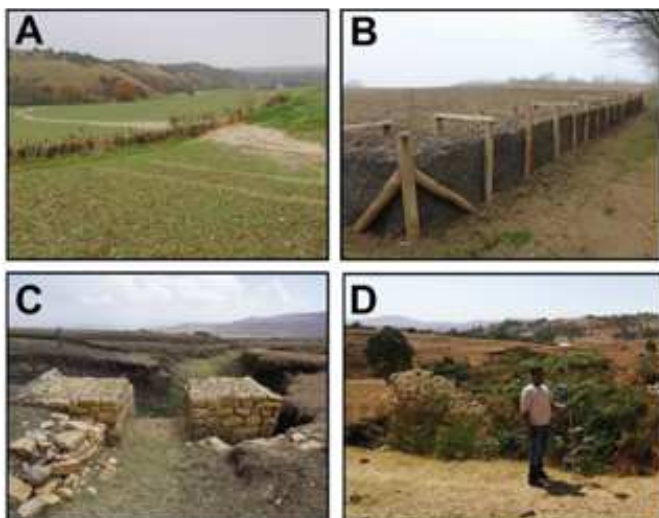
Figure 1: Examples of gully prevention and rehabilitation measures discussed. A: fascine (willow) (N France), B: woodchips barrier (W Belgium), C: in-channel check dams (bypassed) (N Ethiopia), D: revegetation (NW Ethiopia).
