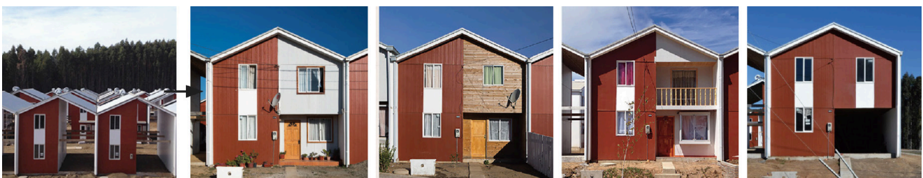
[Figure 3] The same house becomes many houses: Open-ended Design through unfinished products
