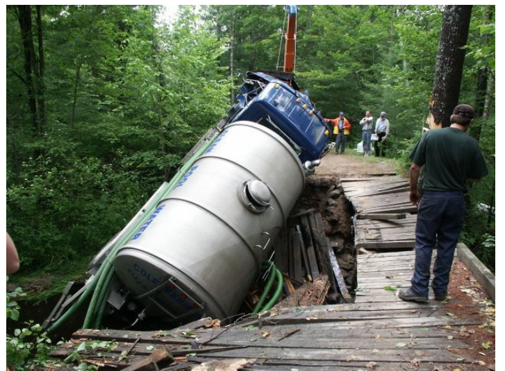
Collapsed bridge with truck in the stream and leaking diesel fuel from its saddle tanks.
