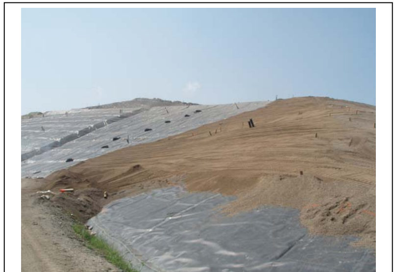
Pine Tree Landfill Cover System Under Construction Hampden, Maine
