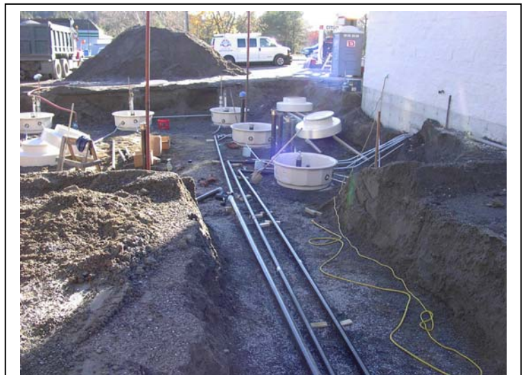
Installation of new petroleum U.S.T.s and piping in Augusta
