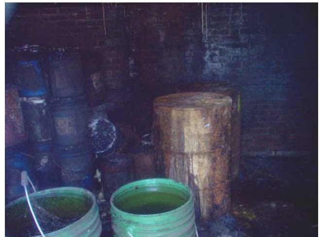
Leaking and corroded containers at a hazardous waste cleanup site in Lewiston (2007)
