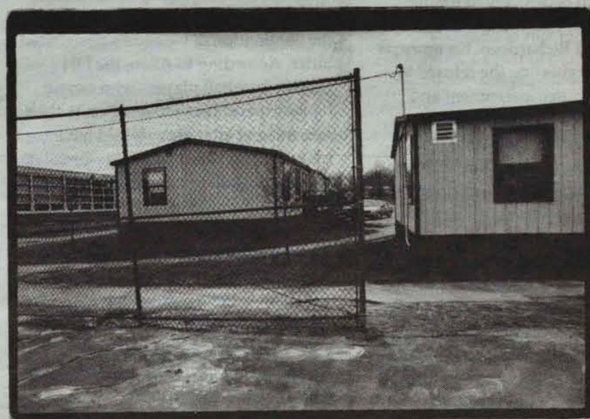
SCHOOL HOUSE: Modular classrooms behind Lyman Moore Middle School handle the overflow of students from a building long outgrown.
