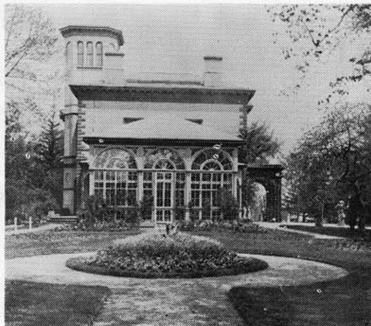
BRAMHALL, John B. Brown’s villa on the Western Promenade.
