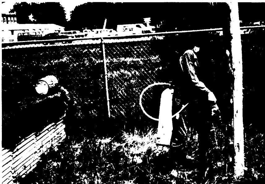
FIG. 3. Application of gelled chloropicrin into pole with a pressurized tank system.
