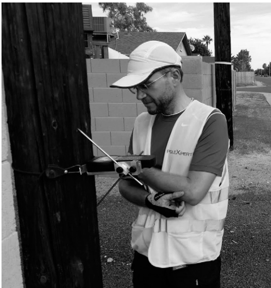
Figure 1. A PoleXpert specialist affixes the PX device, which is used to nondestructively evaluate an in-service wooden utility pole, at approximately 1.22 m above the ground line.
