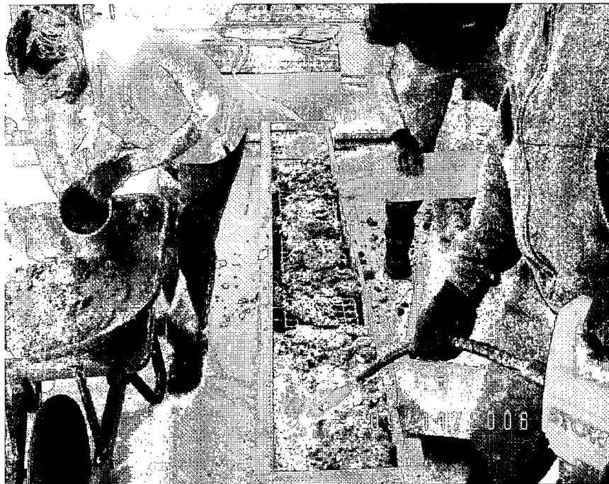
Figure B.4 Pouring the Concrete in Beams.
