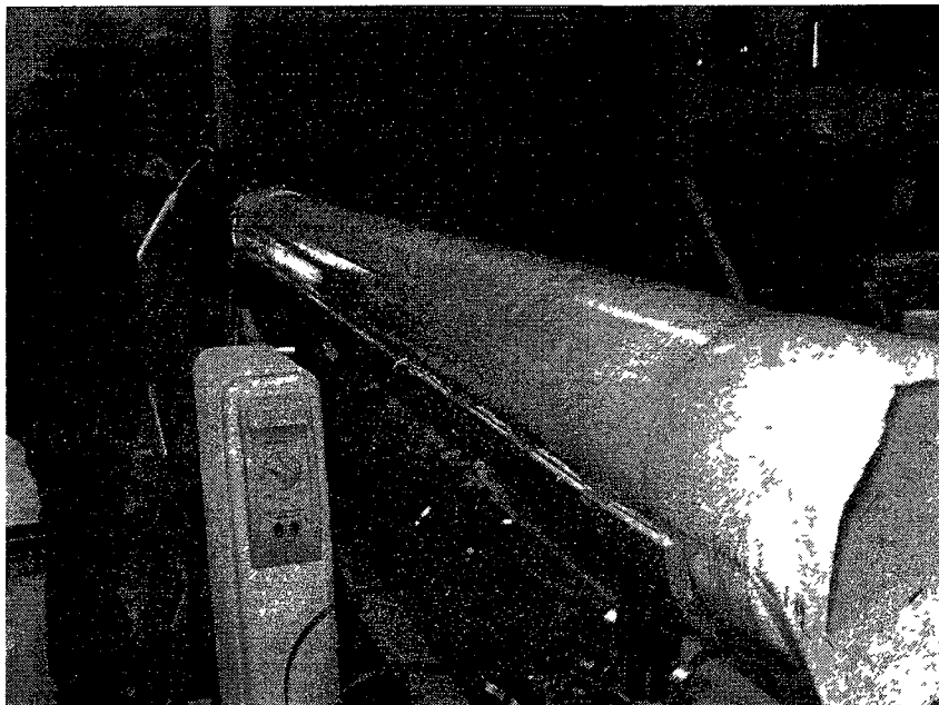
Figure 59: The Finished Product - Cured CIPP Liner
