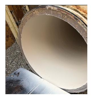
Figure 6-7 Epoxy Coating for the PCCP pipe (ESCS Pipe Coating, 2018)
